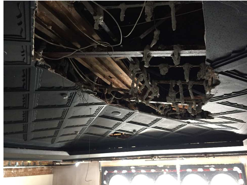
Existing suspended ceiling and roof frame
